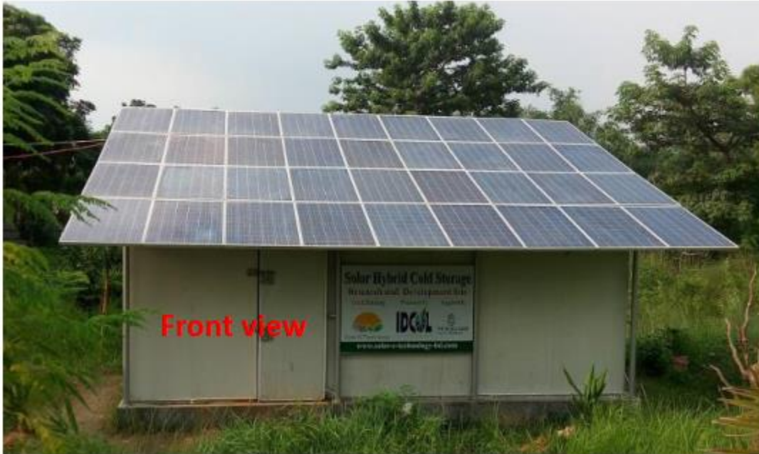
Fig: Solar Hybrid Cold Storage R&D site at Chuadanga
