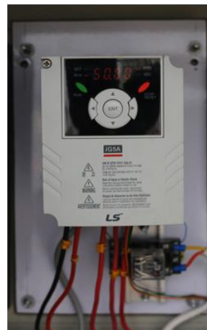
Picture of the inverters used in the cold storage
