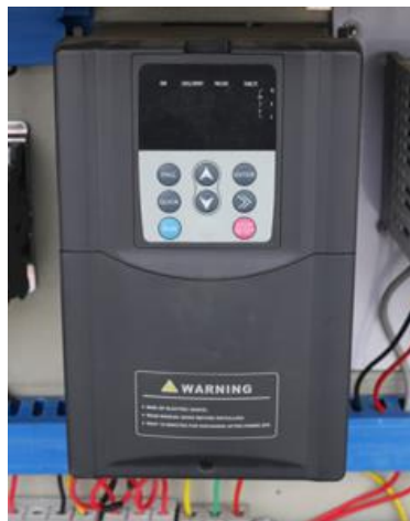
Picture of the inverters used in the cold storage
