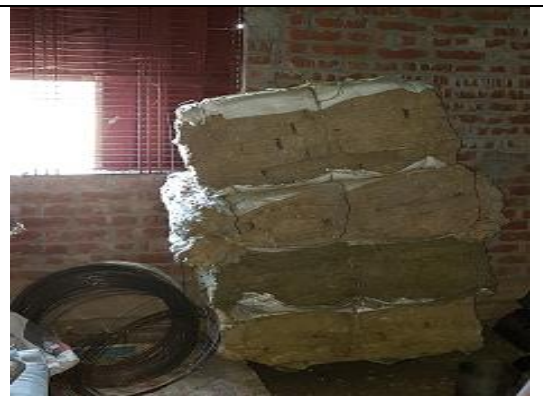
Rockwool storage in open space
