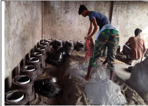
Sand & Cements mixing
