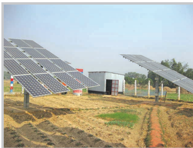
11.2 kw solar irrigation pump of Grameen Shakti at Sapahar, Naogaon
