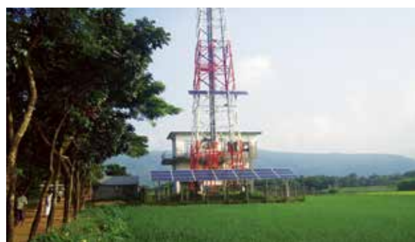
Solar powered BTS of Grameenphone Limited
