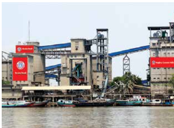
Energy-efficient Vertical Roller Mill (VRM) based Meghna Cement Mills at Mongla, Bangladesh with 9,800 MT per day capacity operating under the brand name “King Brand Cement”
