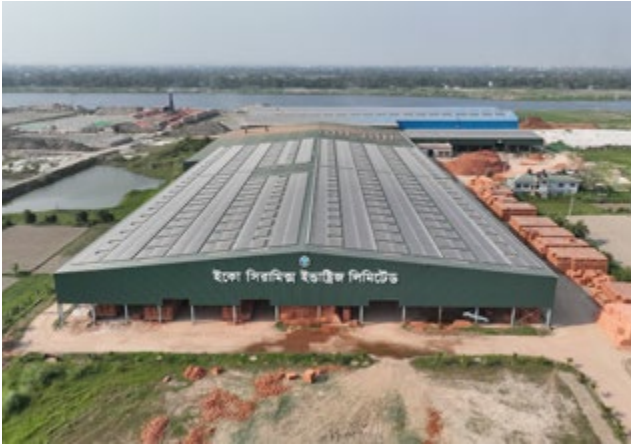
6 MWp rooftop solar project on the rooftops of GPH Ispat Ltd. and Eco Ceramics Industries Ltd. by GPH Renewable Energy Ltd.
