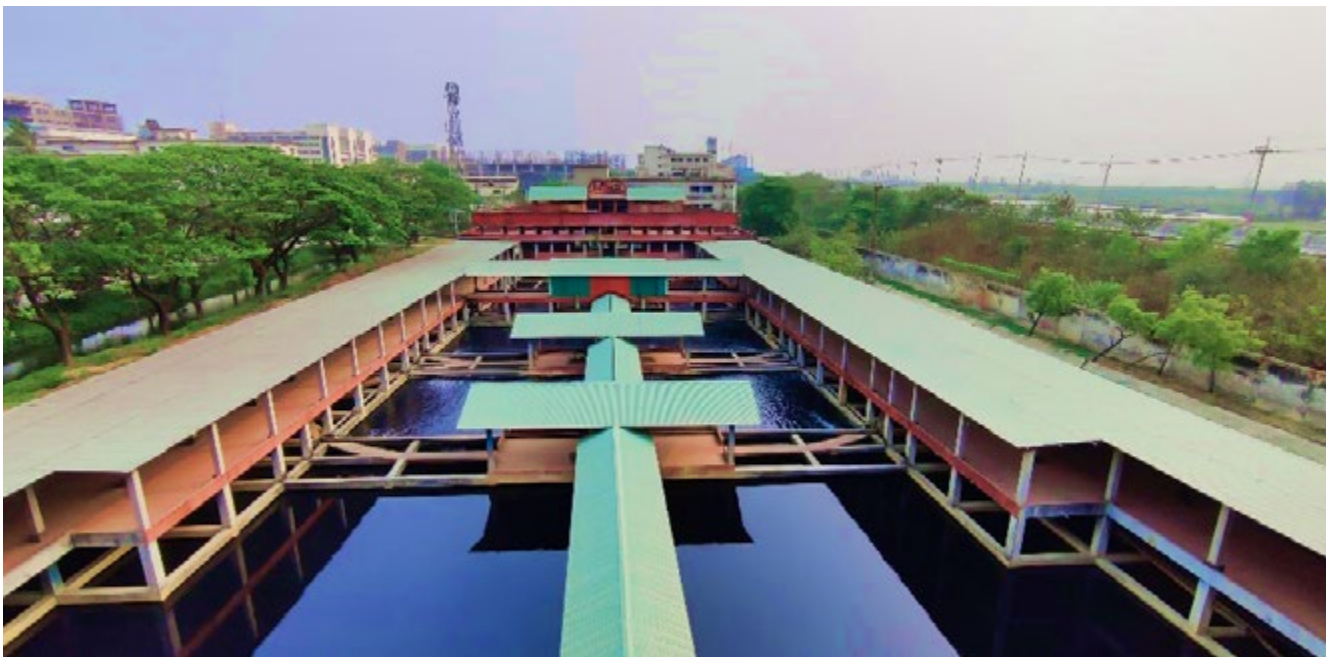
Chittagong Waste Treatment Plant Ltd.
