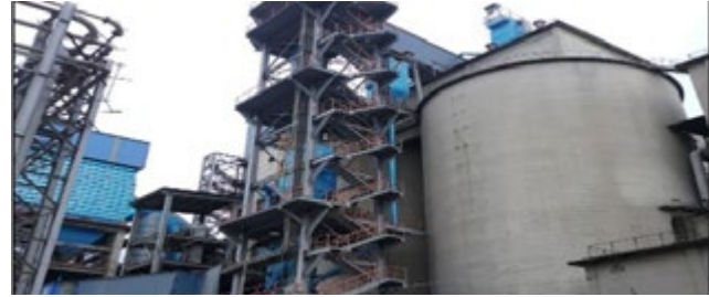
Clinker Feeding System
