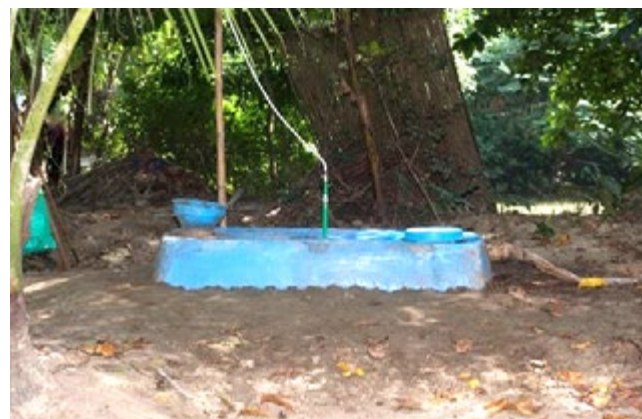
Prefabricated bio-digester based on fiberglass.
