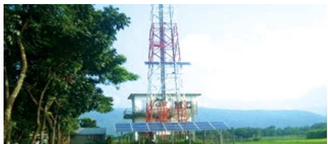
Solar powered BTS of Grameenphone Limited
