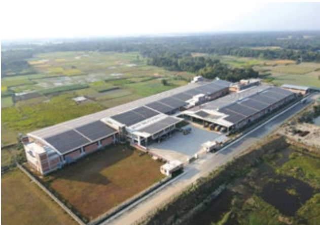
2.80 MWp rooftop solar project on the rooftops of AKH Knitting and Dyeing Ltd.
