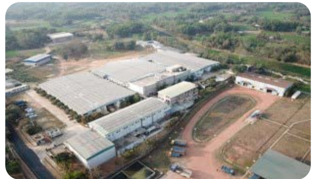
1.49 MWp rooftop solar project of Naafco Pharmaceuticals Ltd.
