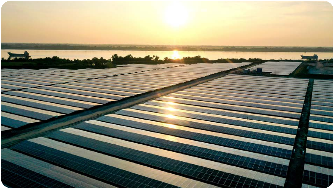
Approved financing to Energon Renewables, country's 2nd largest Solar Park with a 100 MW (AC) capacity located at Mongla, Bagerhat
