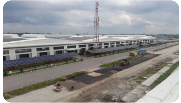
3.32 MWp rooftop solar project of Walton Group
