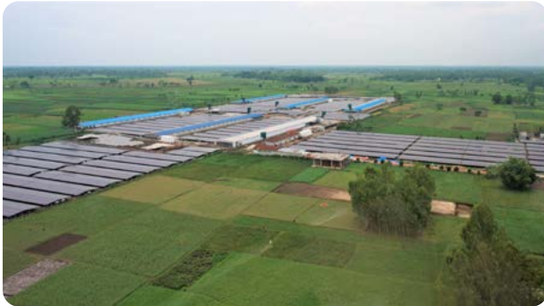
Financed 8 MW (AC) Solar Grid-tied Project of Sympa Solar Power Ltd. located at Tetulia, Panchagarh
