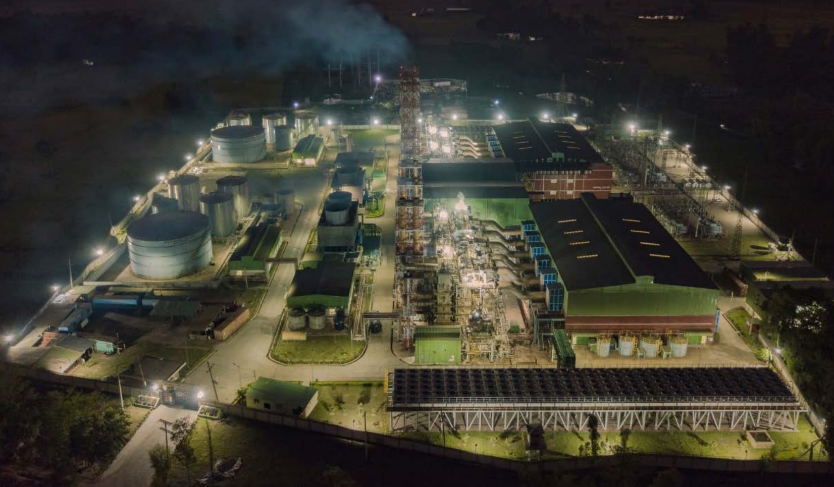
113 MW HFO fired power plant of Confidence Power Bogura Ltd.
