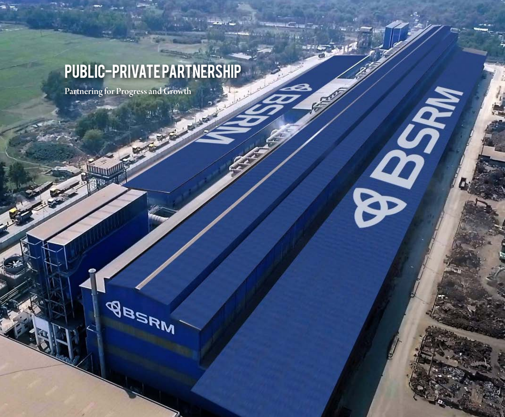
Environment Friendly Steel Manufacturing Plant of BSRM Steels Ltd.
