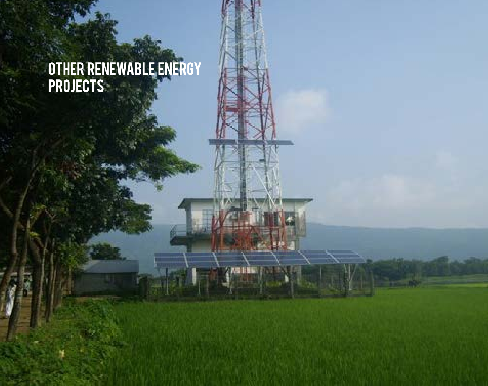
Solar powered BTS of Grameenphone
