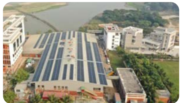
428.22 kWp rooftop solar project of K. A. Design Ltd.
