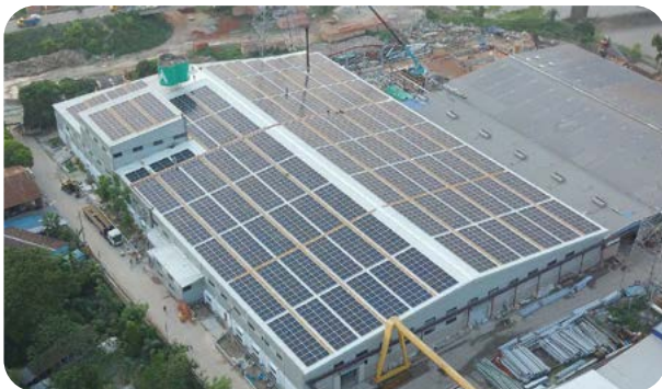
2.00 MWp rooftop solar project of Akij Polymer Industries Ltd.
